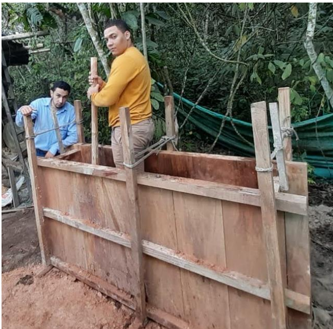
Figure 2. Wooden formwork.
