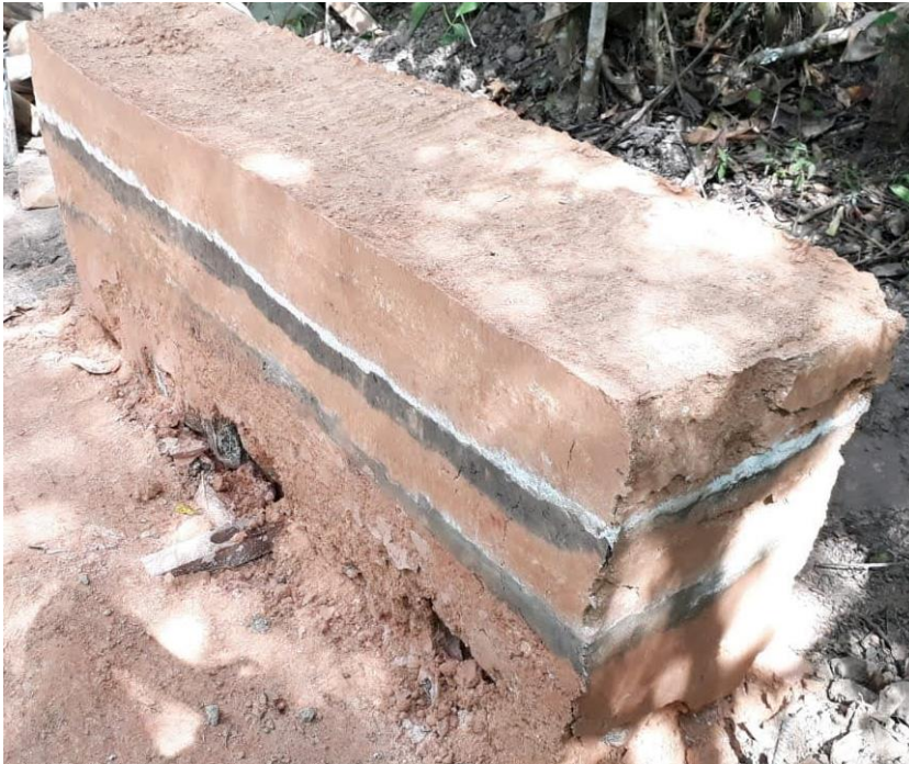
Figure 5. Tapia Wall
