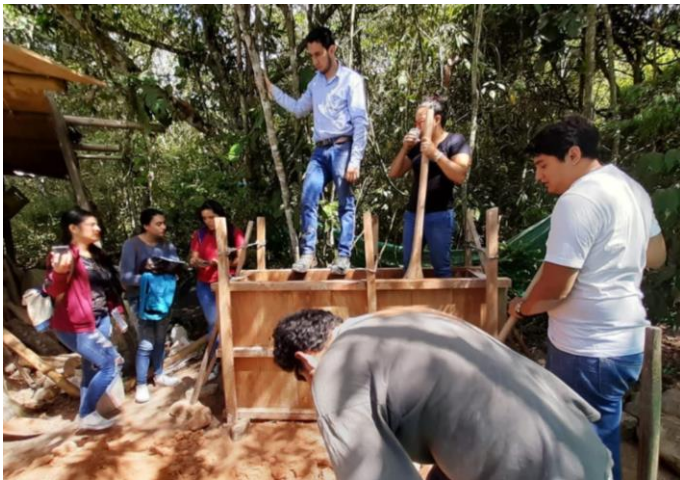
Figure 4. Tamped Tapia Wall
